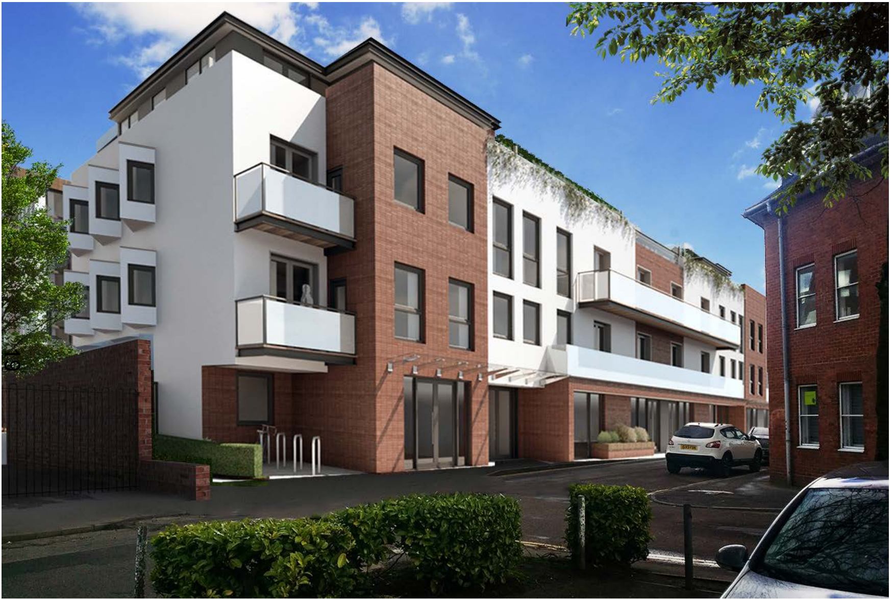
Photomontage of building within Collins Street, corner of Chapel Street (N.B Large sycamore to LHS of picture is closer to wall and much larger in reality with branches overhanging site).
